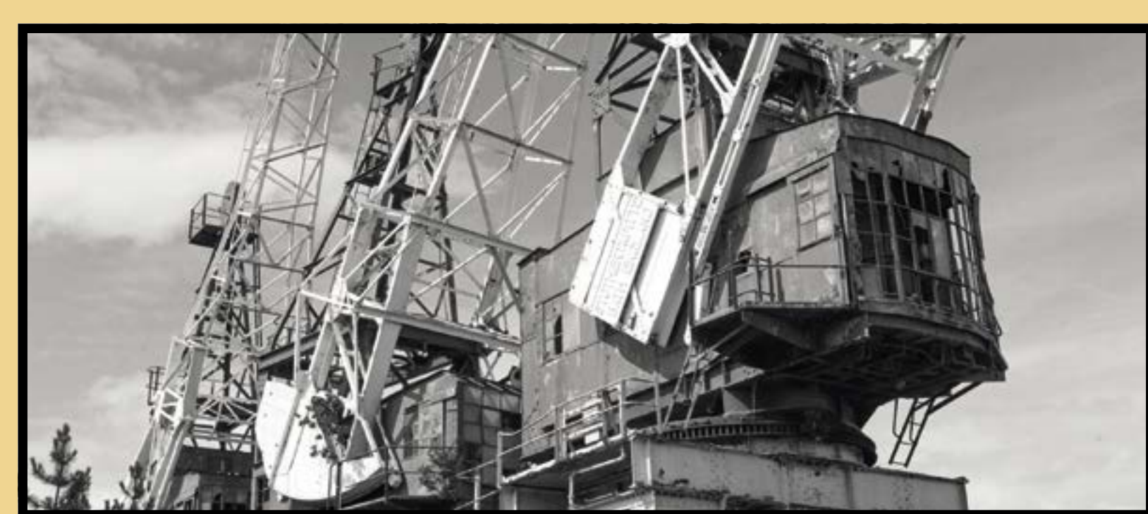
GRAND TRUSSES / BRACING
