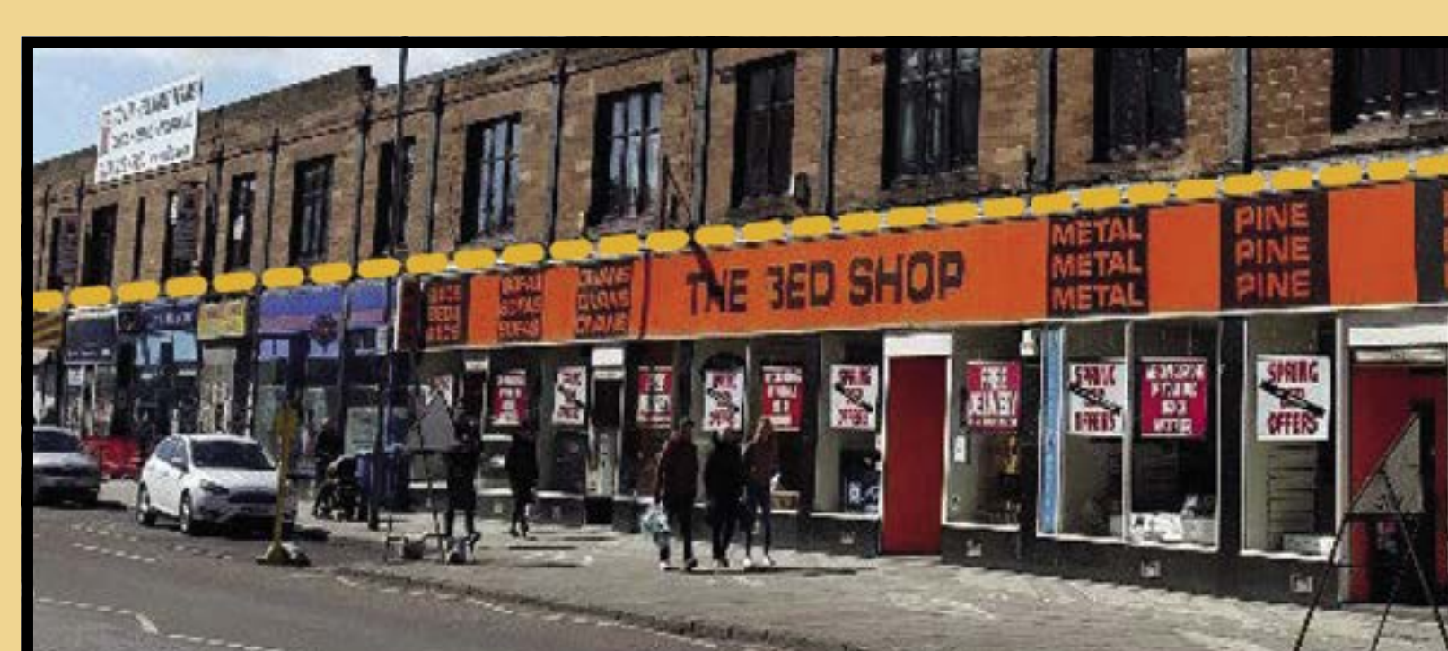
VARIED SHOP FRONTAGE
